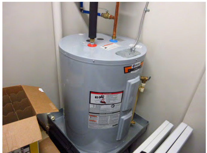
VIEW OF DOMESTIC WATER HEATER
