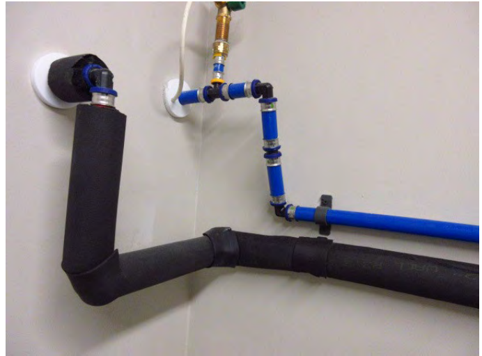
VIEW OF DOMESTIC WATER PIPING
